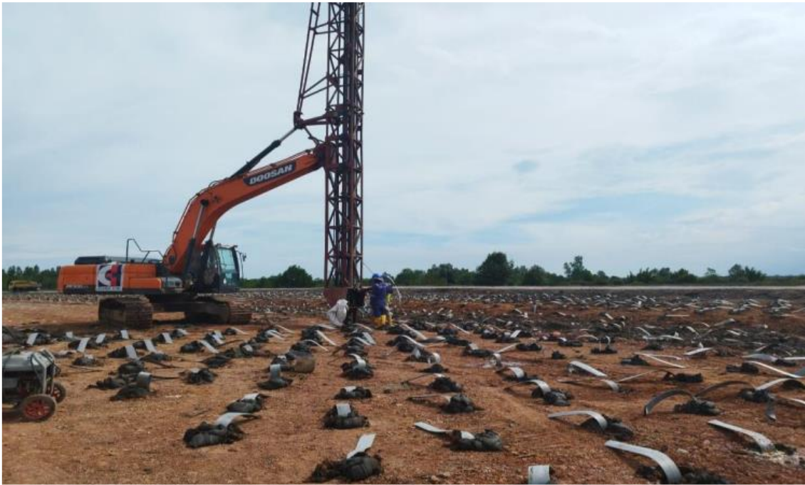
Gambar 3. Proses Pemasangan Mesin Prefabricated Vertical Drain (PVD) .
