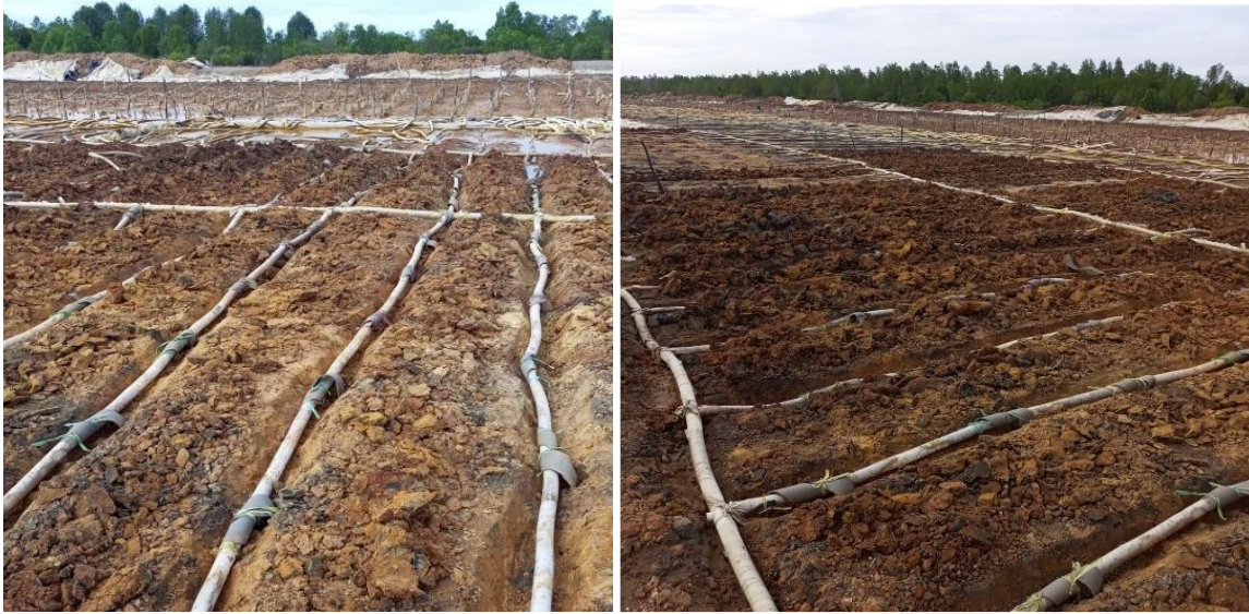
Gambar 4. Perforated Horizontal Drain (PHD) .
